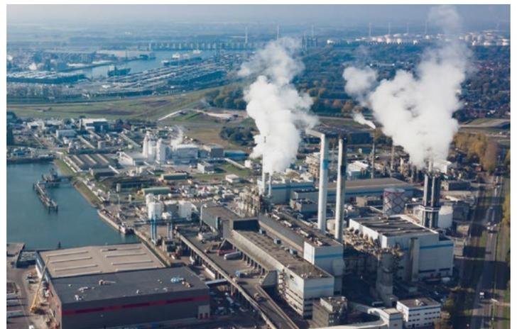
In the E-thor pilot project, a 5 MW electrolyser is at the heart of a promising business model. It is powered by electricity from AVR's waste processing plant, and the oxygen produced alongside hydrogen is used by chemical company Tronox to manufacture pigments. The hydrogen can be used as fuel or feedstock, or can be combined with CO or CO<sub>2</sub> to produce methanol or other chemical products.
